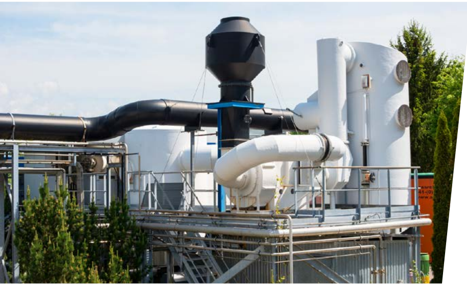
RECYCLING AT BRENNTAG SWITZERLAND: Solvents in particular can be processed in the company's own recycling plant and thus are ready for further use.
